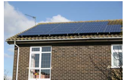
Figure 6.5. Solar photovoltaics: data from a 25\text{-m}^2 array in Cambridgeshire in 2006. The peak power delivered by this array is about 4 kW. The average, year-round, is 12 kWh per day. That's 20\text{ W} per square metre of panel.
