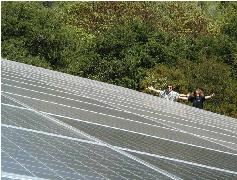
Figure 6.6. Two solar warriors enjoying their photovoltaic system, which powers their electric cars and home. The array of 120 panels ( 300\text{ W} each, 2.2\text{ m}^2 each) has an area of 268\text{ m}^2 , a peak output (allowing for losses in DC-to-AC conversion) of 30.5 kW, and an average output – in California, near Santa Cruz – of 5 kW ( 19\text{ W}/\text{m}^2 ). Photo kindly provided by Kenneth Adelman.
