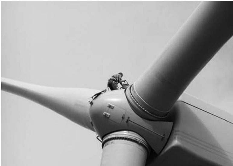
Figure 7.3. Maintenance on a Windmill
